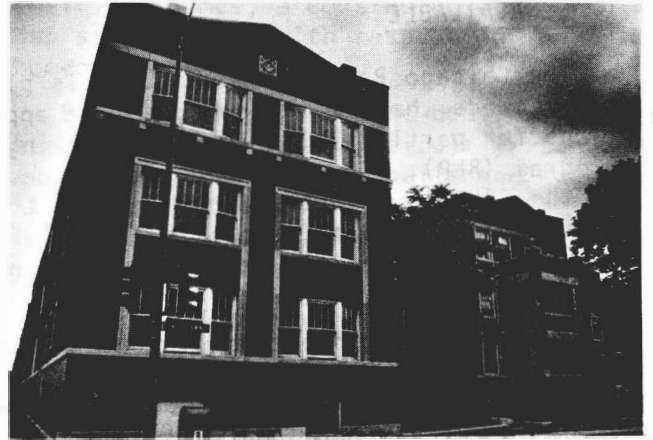
This Woodlawn building was scheduled for rehab into 22 cooperative units for low and moderate income families until the Reagan freeze on 312 loan funds stopped processing.
