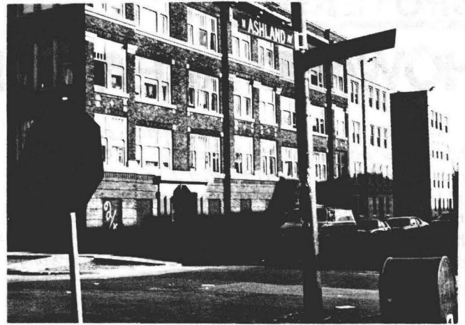
View of two buildings scheduled for rehab by RESCORP/AMOCO partnership in North of Howard area.
