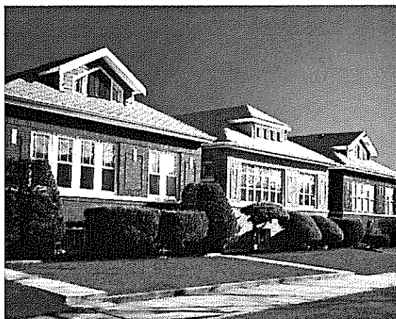
At the expo, owners of bungalows such as these were able to learn about the various resources offered by the City to help rehab and preserve their homes.
