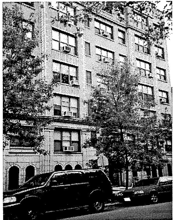
Exterior of Hyde Park Apartments
