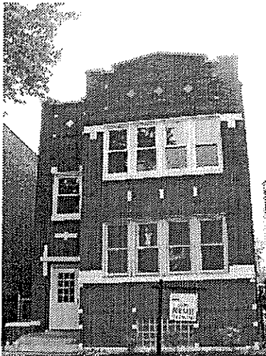
Exterior of recently rehabbed house in the 6100 block of South Fairfield
