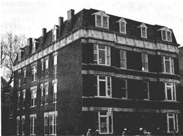
Completed building at 901 West 19th St. Pictured at upper right is Soyla Villicano who served as coordinator of project.
