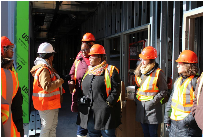
Students tour Altgeld-Murray housing construction site during Project & Construction Management with instructor Angela Hurlock
