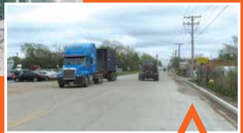
167th Street (CN Terminal/Harvey and South Holland Industrial Districts): Under Construction
