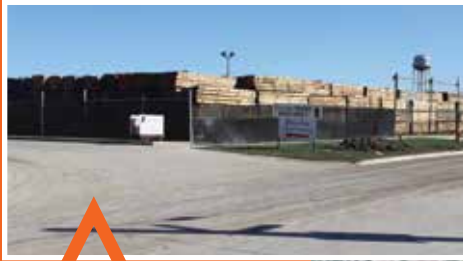
151st Street (Sterling Lumber): Built
