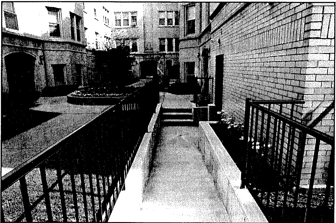
The accessible entrance to Brown and Smith's new apartment.
