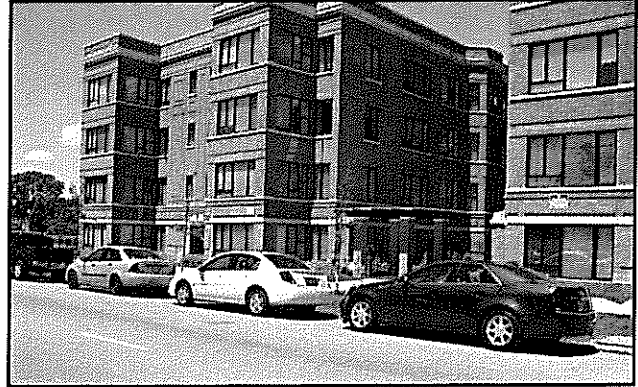
DOH invested loans, Low Income Housing Tax Credits, and donations tax credit in the rehab of Fountain View Apartments.
