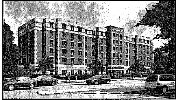
Senior Suites of Kelvyn Park will bring 85 units of affordable senior housing to the Belmont Cragin community and will feature a Department of Senior Services Satellite Center on the first floor.
