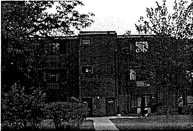
Martin Luther King Jr. Plaza Apartments to receive capital improvements
